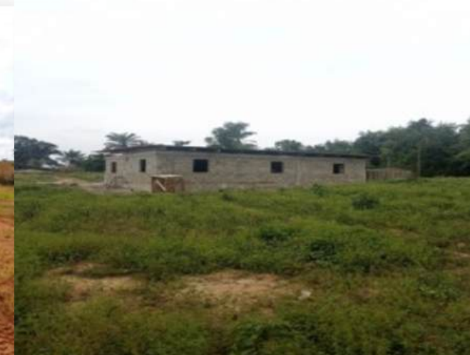
Medical Clinic Construction
