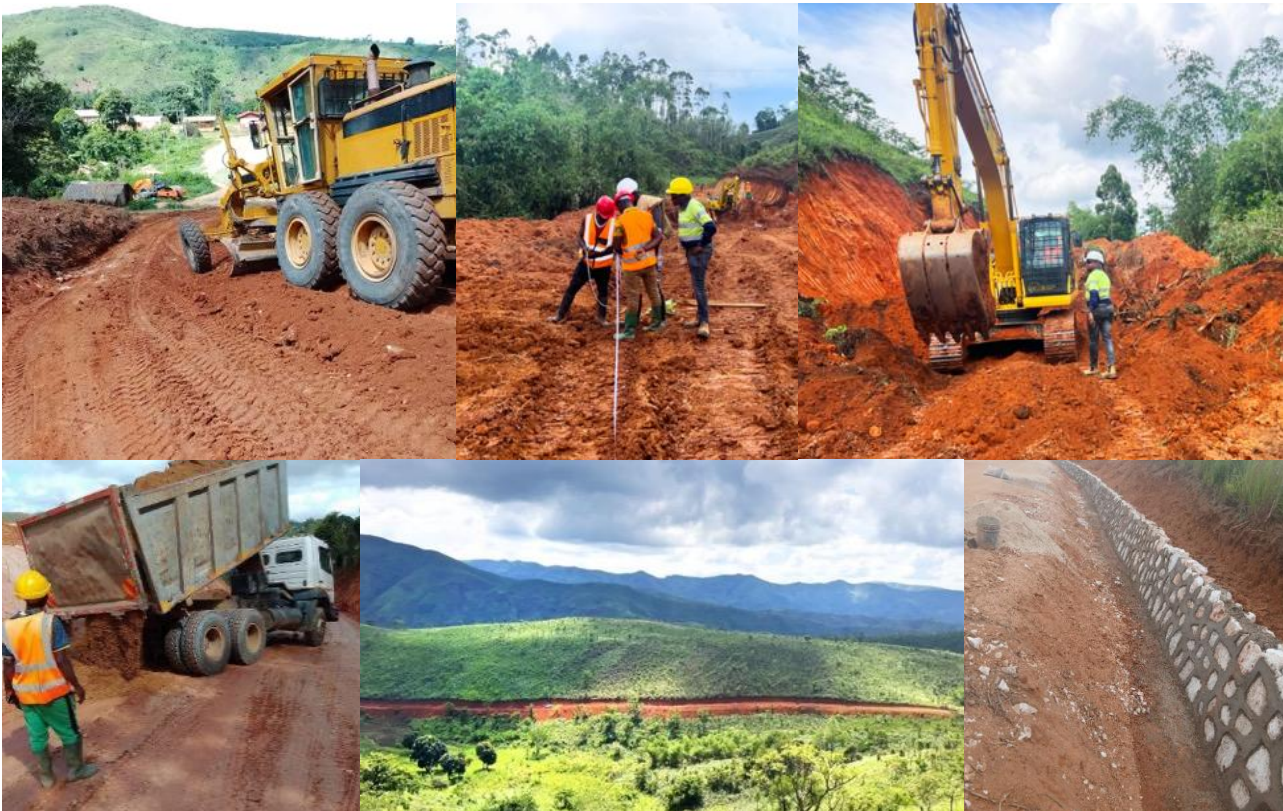
Southern road upgrade
