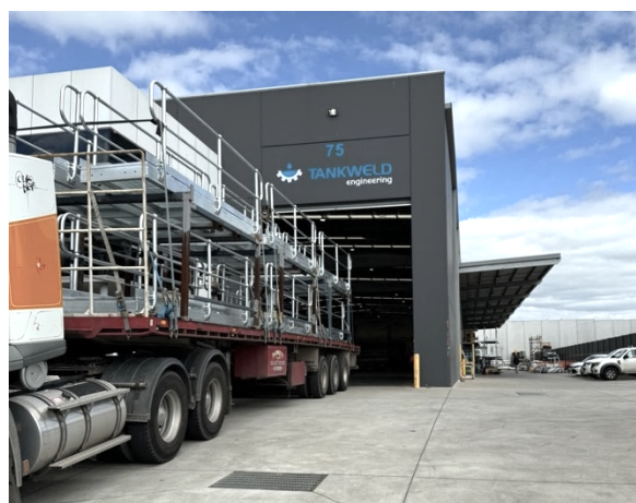
Figure 2b: Finished goods leaving fabrication workshop.
