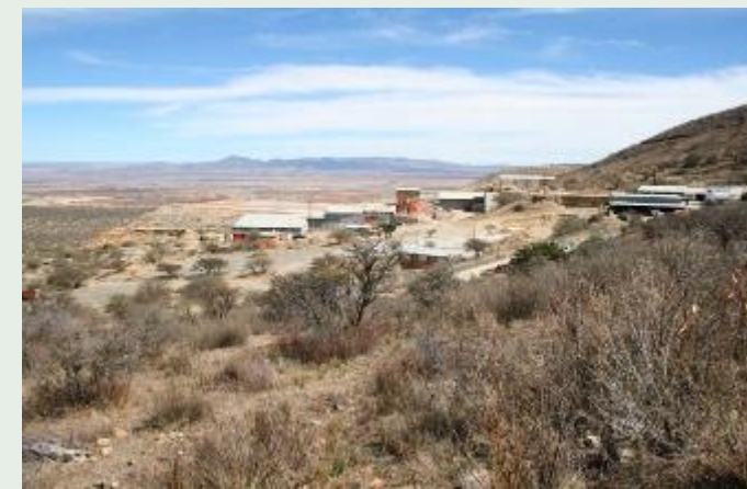
Looking from the west end of the Los Rosarios vein towards the plant, c. 2006
